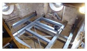
New steel girders span inside the tower, in the 'spare' storey below the old belfry
