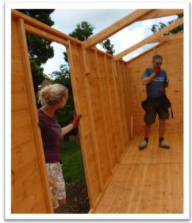
On 26<sup>th</sup> August, Becky, John (of *Sheds from stock*) and Barry gathered in the churchyard to erect a new shed, with Rooster the Ridgeback adding his support. First the sides were erected, then came roof trusses and finally the roof itself. Once roofing felt had been added the only task left to do was to give the structure a protective treatment of Sadolin. The enlarged shed, replacing one that was falling to bits, is necessary for additional storage.
