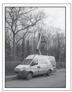
In Whaddon, new poles were placed directly adjacent to old poles, with adjustments made to wires accordingly. Contractors also replaced the previous four electric cables (three-phase and neutral) with one thicker cable). Finally, the old poles were removed.
